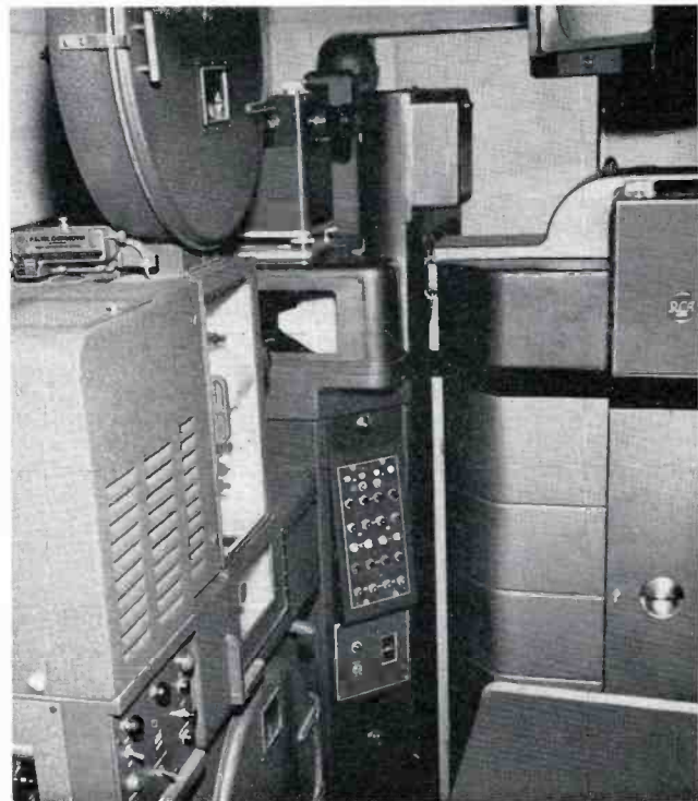
FIG. 9. Complete color and monochrome film system is installed. This includes 35mm film projector, 16mm film projector, and a slide projector. Thus, stock footages and special film shots can be inserted into tv tapes. Equipment is remotely operated from control room.
