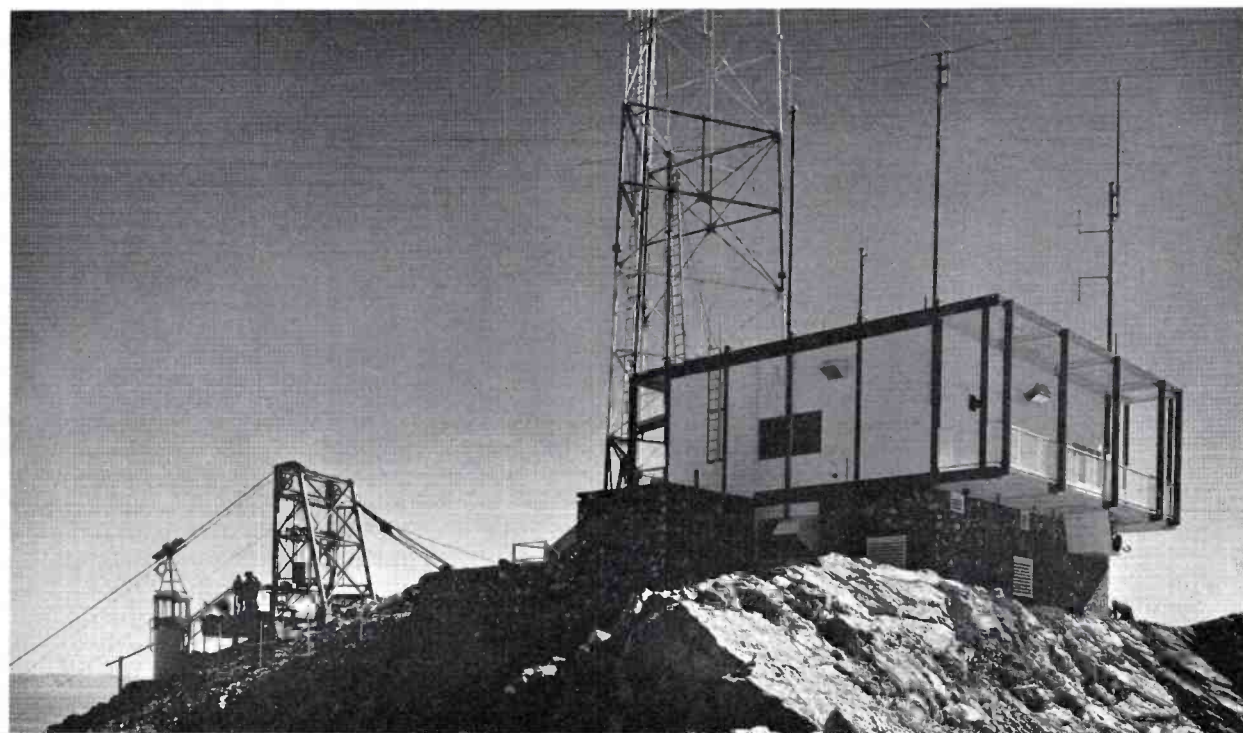
FIG. 3. The peak of the mountain was blasted off to provide room for the building and tower.
