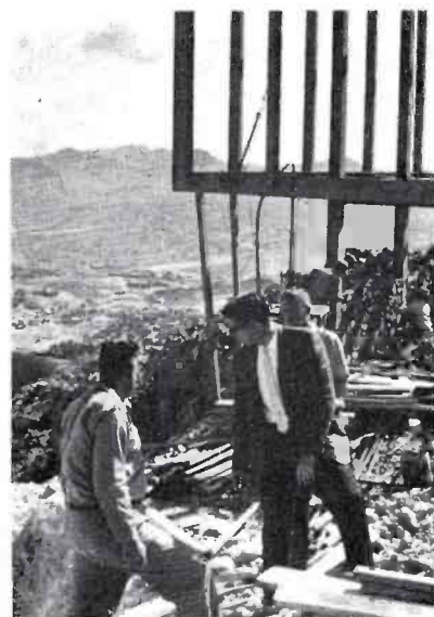
FIG. 4. Typical construction scene while transmitter building was being constructed.
