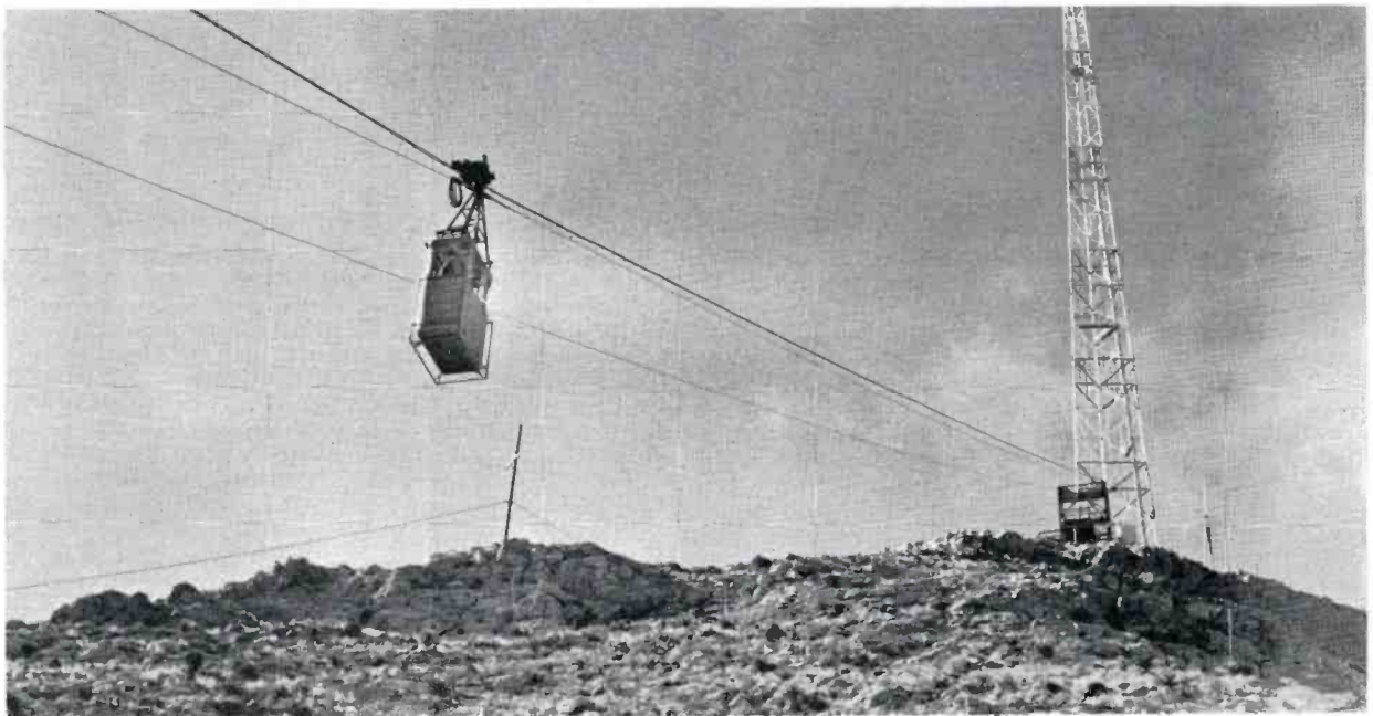
FIG. 6. Riding through the sky to the KTSM transmitter. This tramway is the sole means of transportation for water and other supplies, station personnel and visitors.
